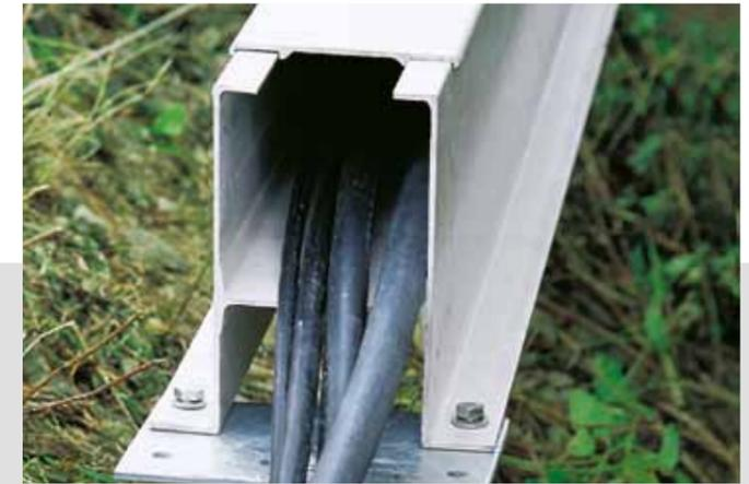
After the insertion of the cables, the lid will be closed with the quick-action fasteners.
