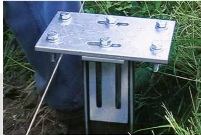
The mounting plates are installed, adjusted and bolted onto the pillars.
