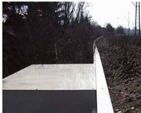
Custom solution: Coupling kit and excess cable kit, pillar-mounted and attached to Vario Top size 1a.
