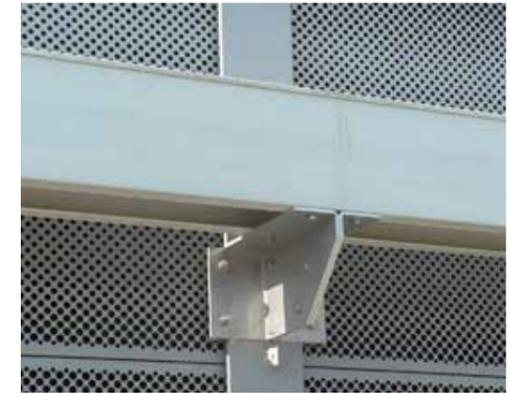
Vario Top size 2 mounted on special mounting brackets along a noise protection wall.
