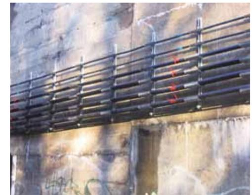
Specific solution used for this particular application: The three parallel cable ducts are mounted on one single pillar only! Custom solution: Cable troughs mounted on C-rails.
