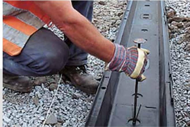
Securing of the cable duct by means of specific ground anchors in accordance with the requirements on site.
