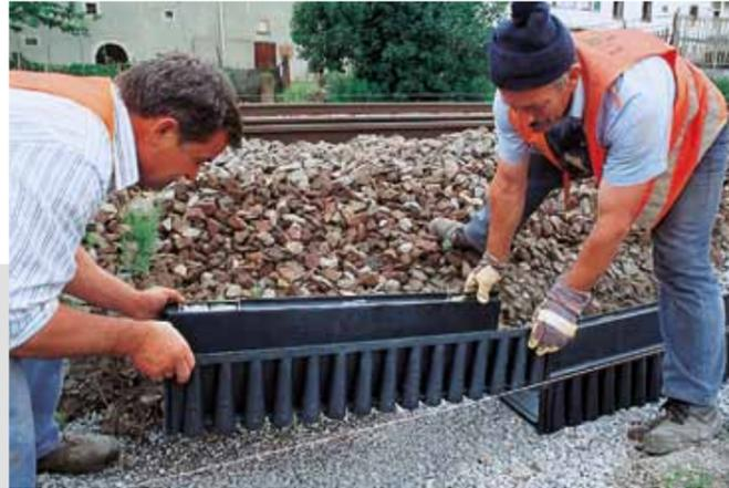
Installation of the ducts in the cable pits prepared beforehand.
