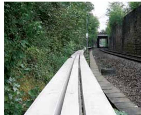
Custom solution using the VARIO TOP pillar-mounted cable duct system consisting of one duct size 1 and two ducts size 2.
