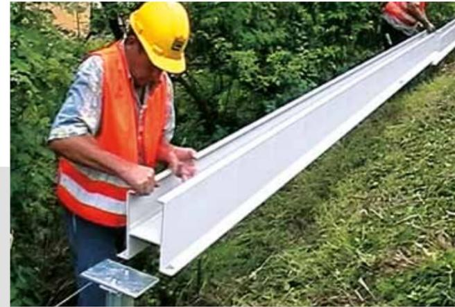
The cable ducts are positioned and bolted onto the mounting plates.
